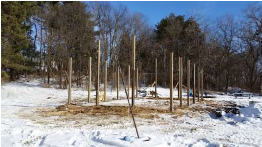
The new RRLC Shelter with all posts set!
